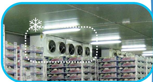
By cold-storage chamber we mean a room built using thermal insulating material and which is used to preserve perishable goods by means of refrigeration. Immediately after collection, fruit and vegetable must be put in cold storage to prevent rot and decay.
